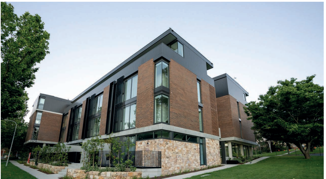
MICA (Middle of Campbell) – Rooftop, terrazze e aree esterne Campbell, Australia Pedestal System – New Maxi NM
